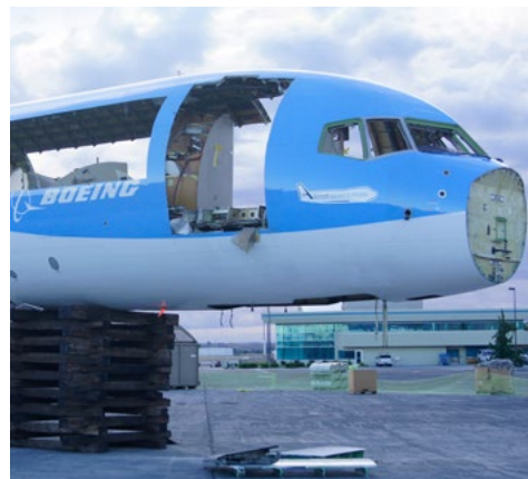
Dismantling equipment for recycling.
