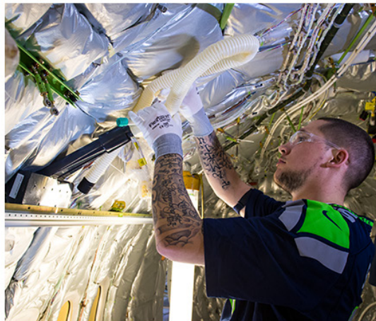
Boeing is implementing a lighter, simpler air distribution system in the 737 cabin.
