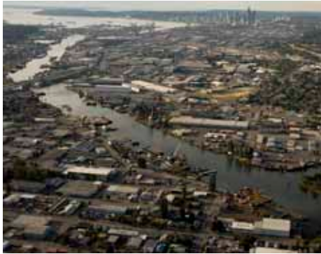
PHOTO: LOWER DUWAMISH WATERWAY GROUP, USED WITH PERMISSION Boeing intends to restore shoreline and create habitat for migratory salmon on our property along the Duwamish, an industrial waterway in Seattle.
