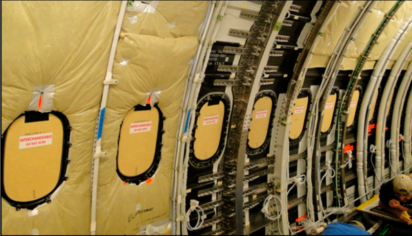
Interior Skin w/ Insulation Blankets
