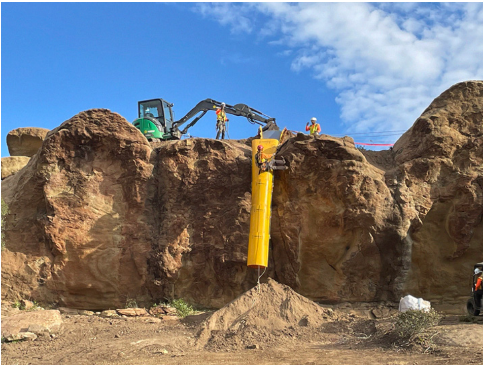
The DTSC-ordered cleanup of the Sage Ranch Shooting Range will remove an additional 15,000 cubic yards of soil
