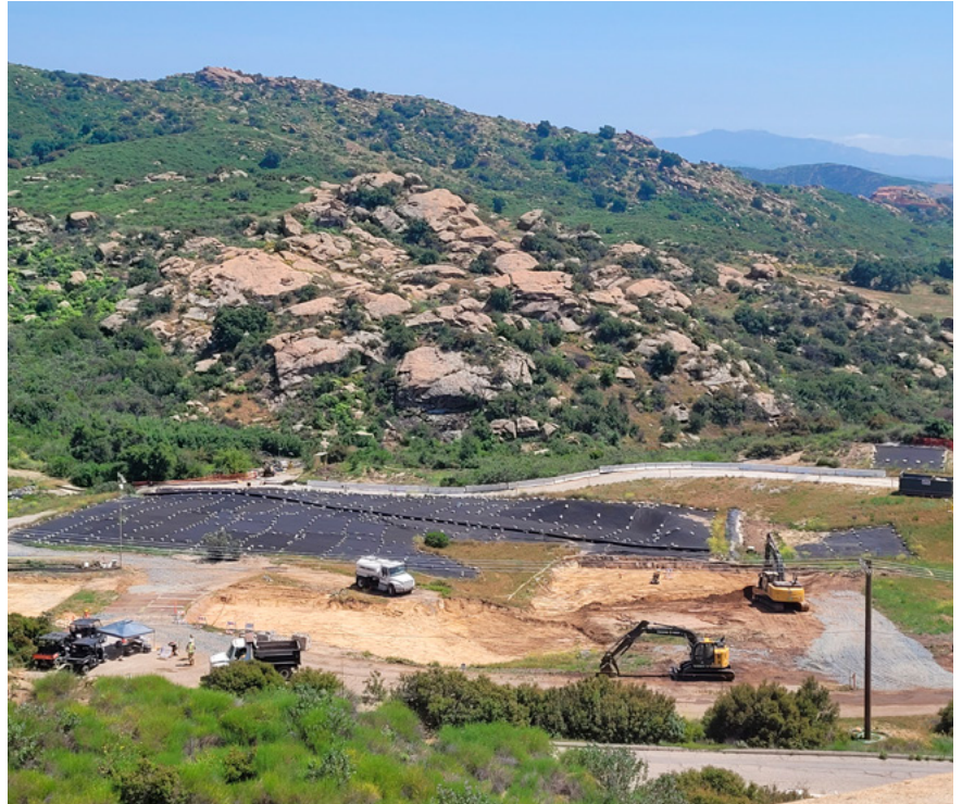
The DTSC-ordered cleanup of the Area I Burn Pit will remove an additional 10,000 cubic yards of soil
