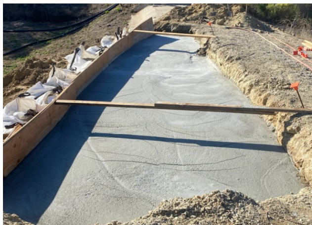
2022: R1 Pond Berm Repair
