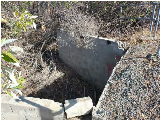
Figure 10. Alternate View of Culvert
