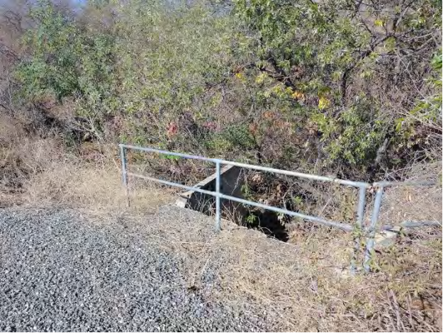
Figure 9. Culvert under Valley Circle Blvd
