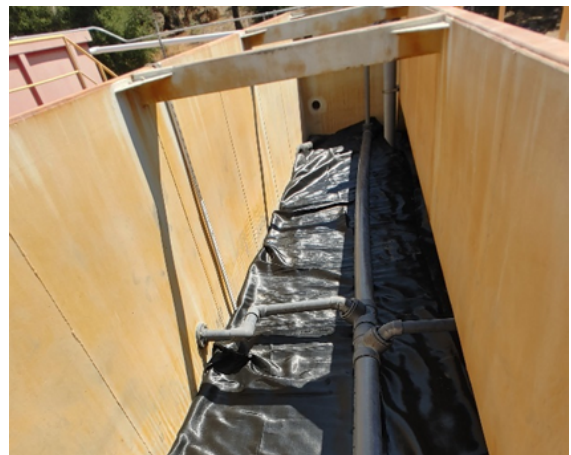
2021: Outfall 009 ELV Treatment BMP Media Filter Reconstruction
