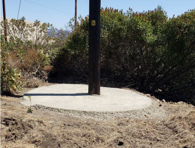
2019: Area II Utility Pole Vegetation Clearing and Soil Base Stabilization
