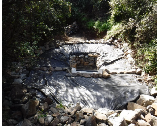
2020: Outfall 009 CM-3 Check Dams Added and Filter Media Reconstruction
