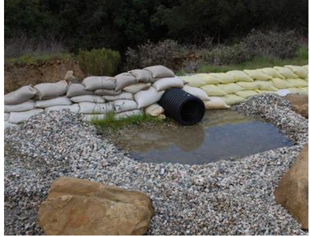
2013: LOX Sandbag Berms and Slope Drains
