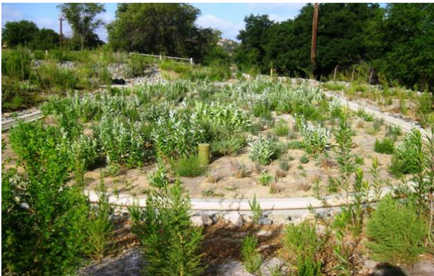
2013: Lower Parking Lot Sedimentation Basin and Biofilter
