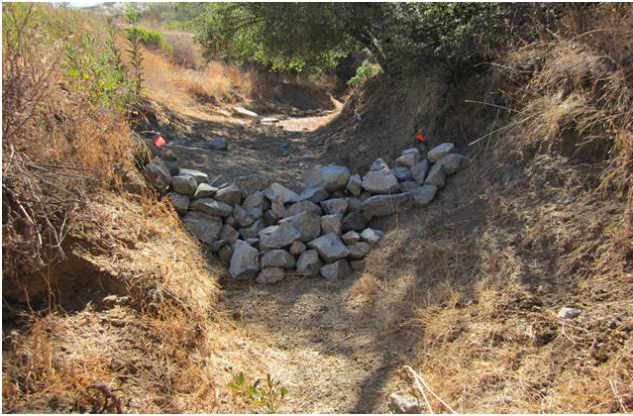
2012: Northern Drainage Restoration Measures
