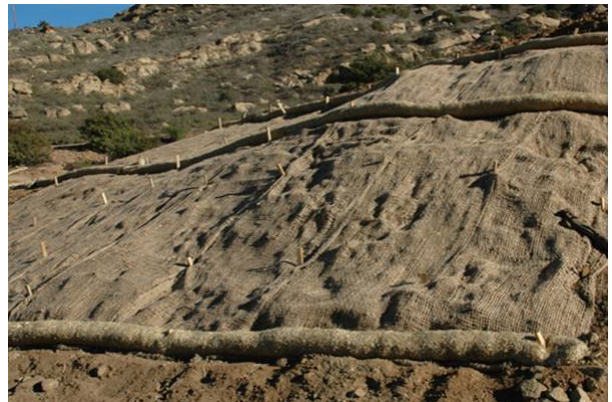
2013: Outfall 009 Watershed ISRA Excavations
