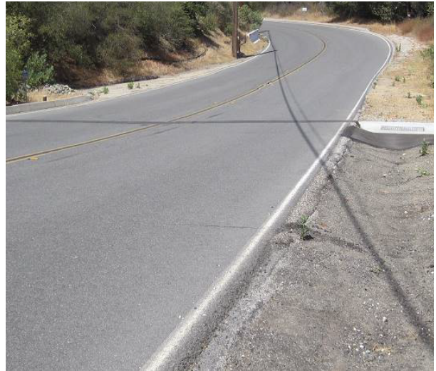
2017: Roadway Diversion to CM-1
