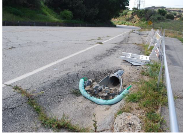
2017: Administration Area Weighted Wattle and Riprap at Culvert Inlet
