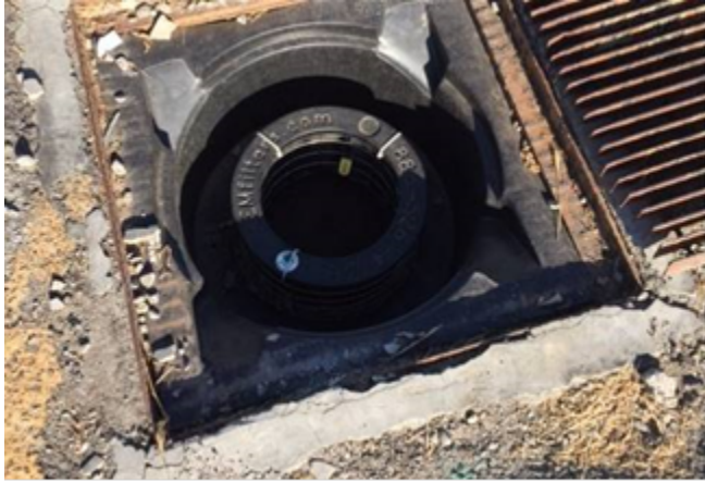
2017: Administration Area Inlet Filter (Filter Basket)
