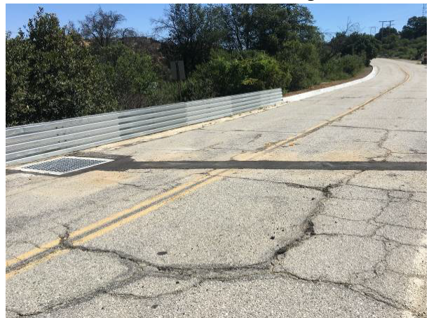
2017: Roadway Diversion to CM-3
