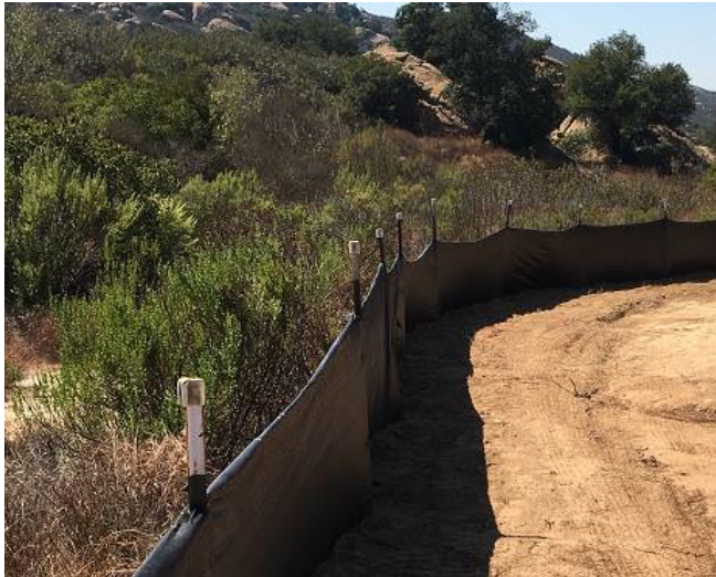
2017: Enhanced Erosion and Sediment Controls in Former Shooting Range Area
