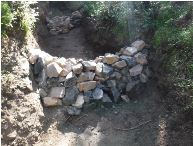
2020: Outfall 009 CM-3 Check Dams Added and Media Filter Reconstruction
