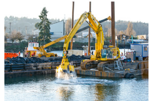
Boeing completed the first phase of removing contaminated sediment and replacing it with clean sand along a half-mile stretch of the Lower Duwamish Waterway. (Boeing photo)
