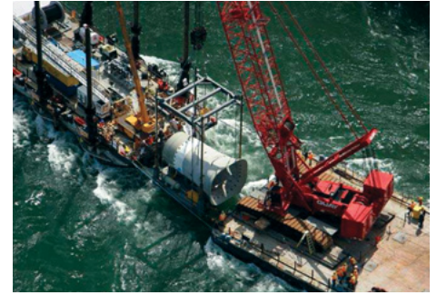
A hydrokinetic turbine is readied for placement in the St. Lawrence River near Montreal, Canada. Boeing and Canadian firm Renewable Energy Research are collaborating on expanding the use of this new source of hydroelectric power. In January 2013, Boeing and RER signed a memorandum of understanding with the government of Quebec to install a six-turbine pilot project in the St. Lawrence River. The turbines provide consistent power without disrupting the river flow or surrounding natural habitat. (Boeing photo)
